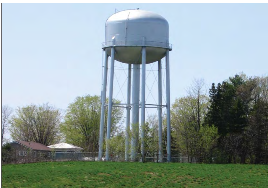
The Village of Sandy Creek and Village of Lacona Joint Water works owns 65 acres of public use land immediately to the south of the Hanson Aggregate industrial land in the Village of Lacona
