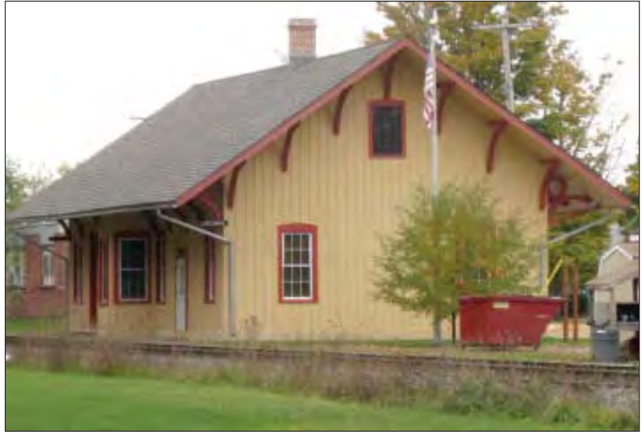
Former New York Central Railroad Station, Park Street in the Village of Lacona, built in 1890.
